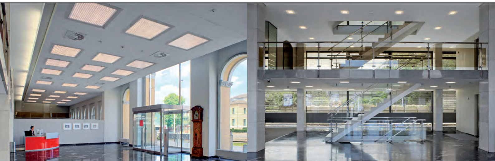
Fig. left Module Q 400 LED.next luminaires generate a pleasant warm-white light with a high level of colour rendering thanks to their partially diffuse light and the brilliance of the LEDs. This means that, depending on requirements, the luminaire can be used to produce a festive or more functional atmosphere in the large hall of the Nord/LB in Braunschweig. Fig. right The Module Q 64 XL LED.next luminaire was deployed to light the staircases.
